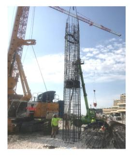
O-cell cage lifting into place for installation into the pile bore
